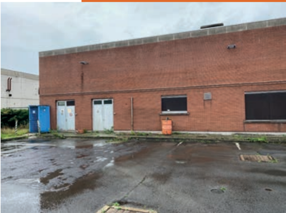
Park Apart — Zwevegem
